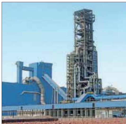
Fig 3 AUMUND conveyor system for DRI in the Middle East, in continuous operation for over 15 years
