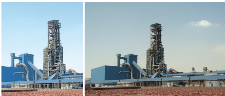
AUMUND conveyor system for DRI in the Middle East - in continuous operation for more than 15 years
