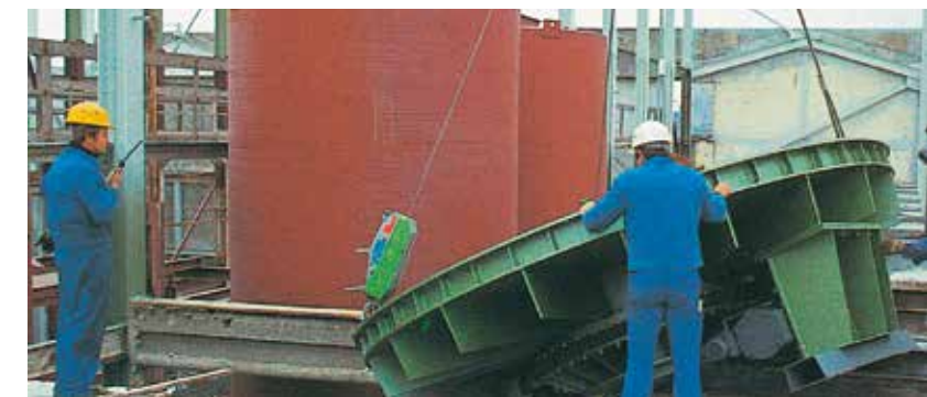
Assembling of CENTREX® bottom in the field
