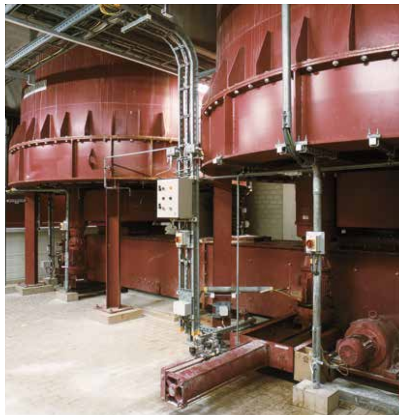
CENTREX® type CTX-AFD with external drive for FGD Gypsum
