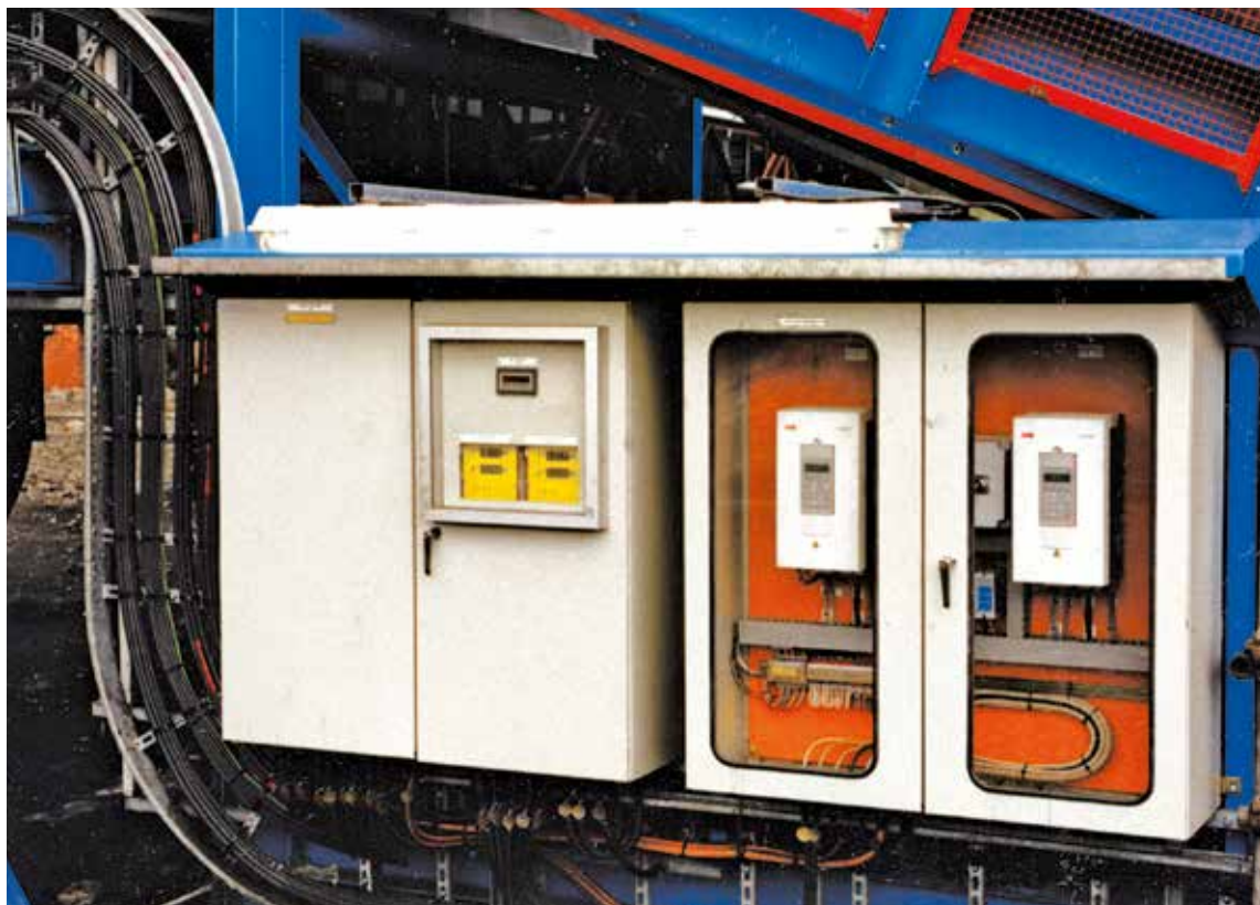
Inverter speed control modules located local to the Samson® MF but linked to a remote control room
