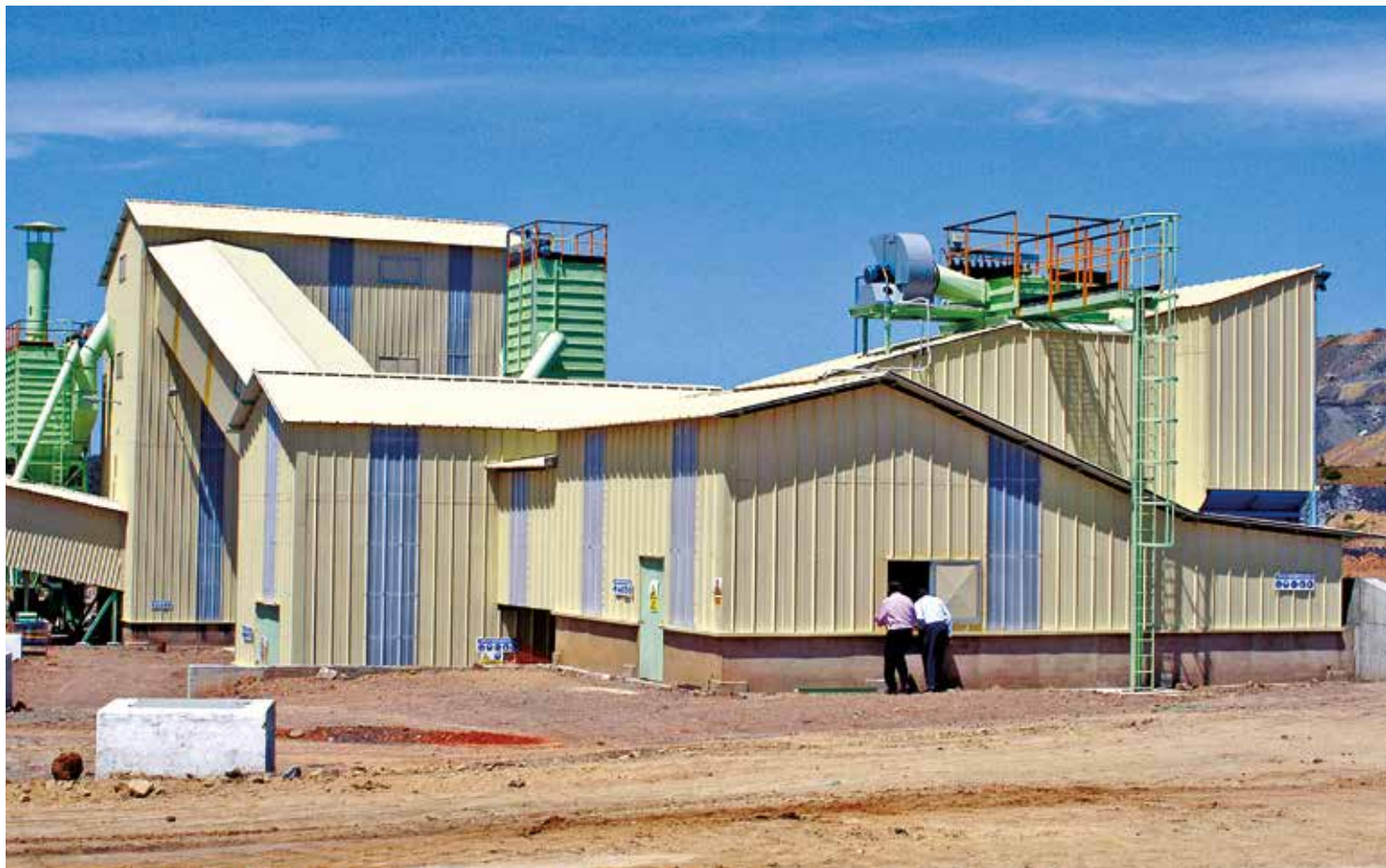
The Samson® MF enclosure integrated to a complete coal preparation plant handling ROM material direct from the adjacent open cast mine
