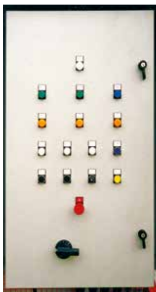
Local cabinet with motor control gear
