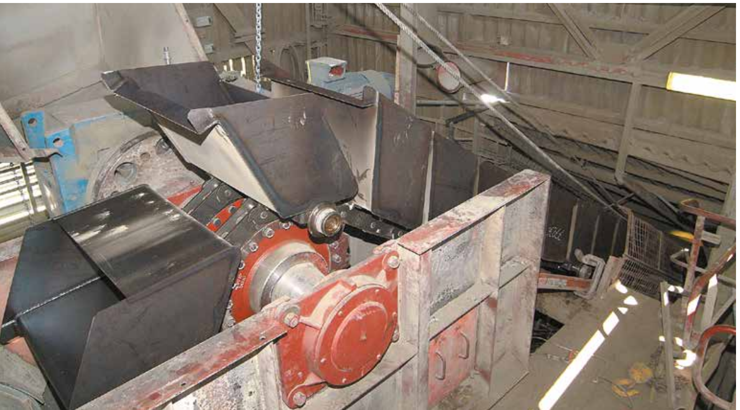
Installation of new bucket strand (example)
