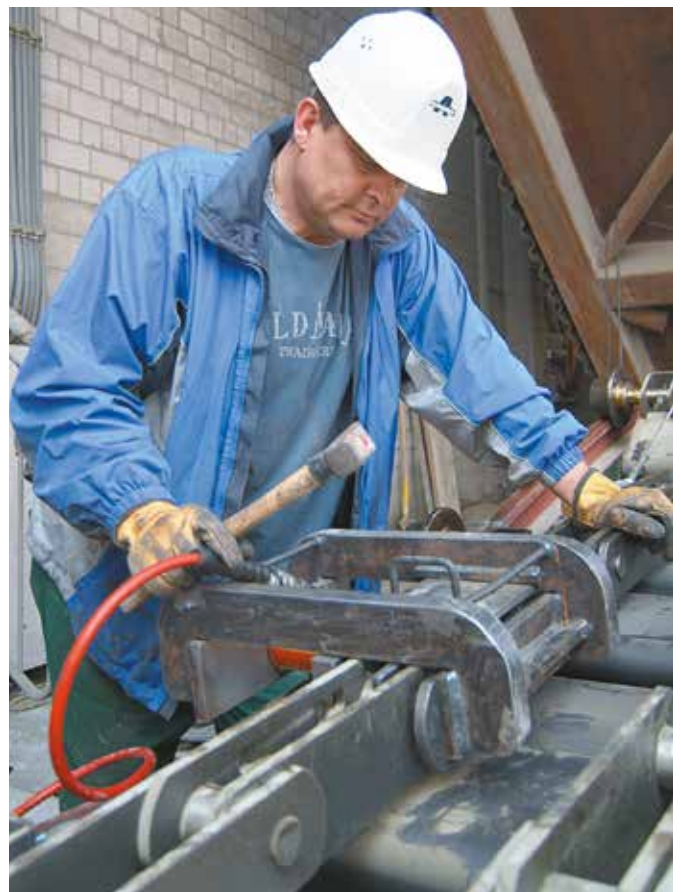
Pre-assembly of chain strands
