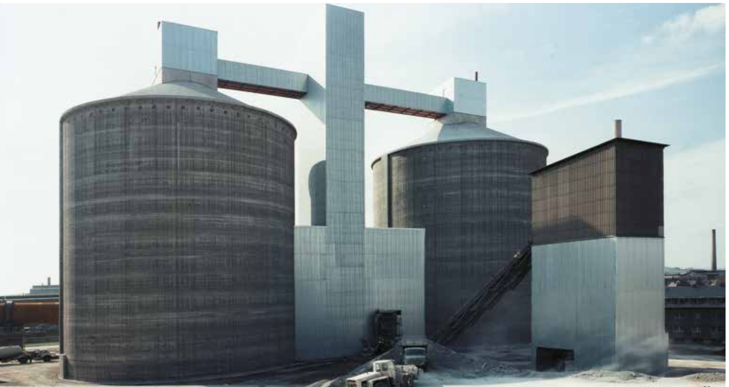
Clinker Silos 2 x 60,000 t (example)
