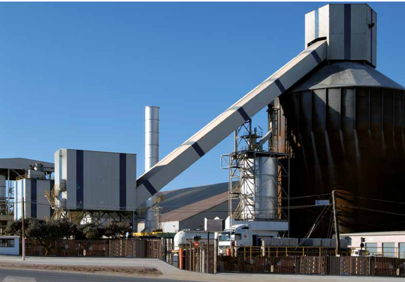
AUMUND Pan Conveyor KZB-Q connecting cooler and silo
