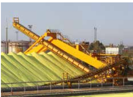
Combined Portal Reclaimer
