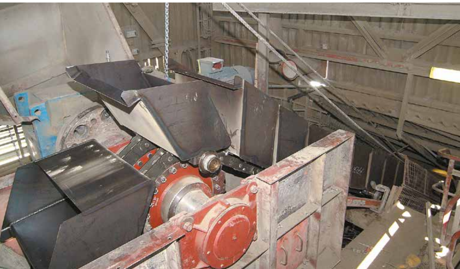
Installation of new bucket strand
