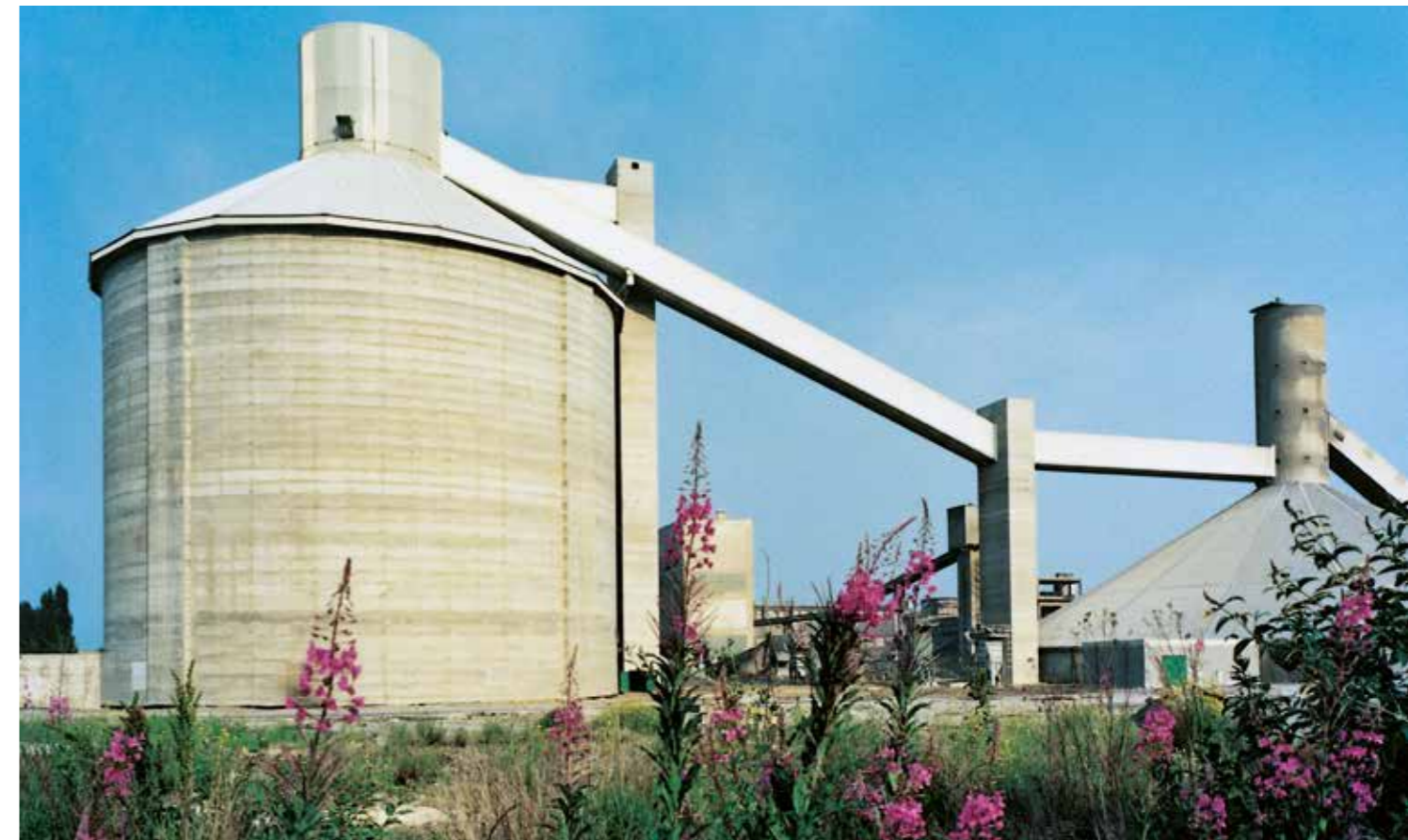
80,000 t silo with steel roof
