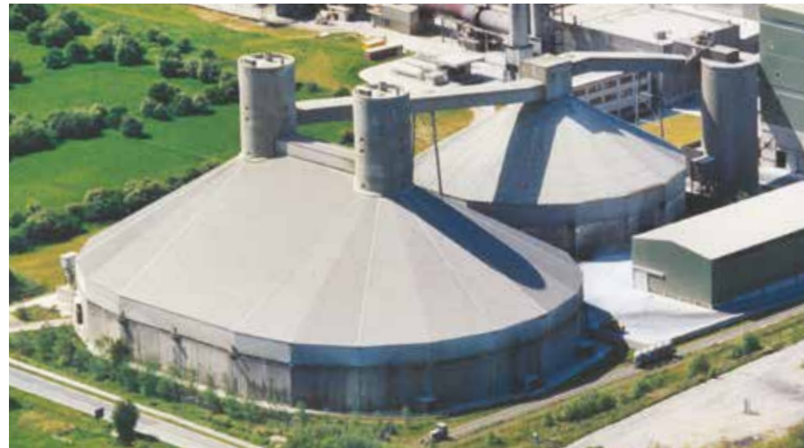
Oval storage hall with internal silos
