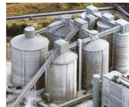
Silo group for different clinker types
