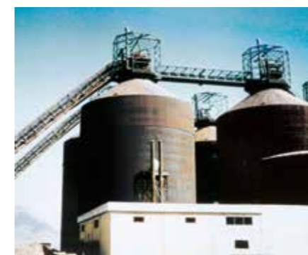
Steel silos, 30,000 t each
