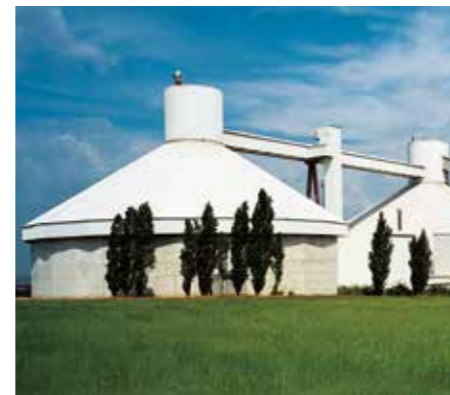
Circular storage hall 60,000 t
