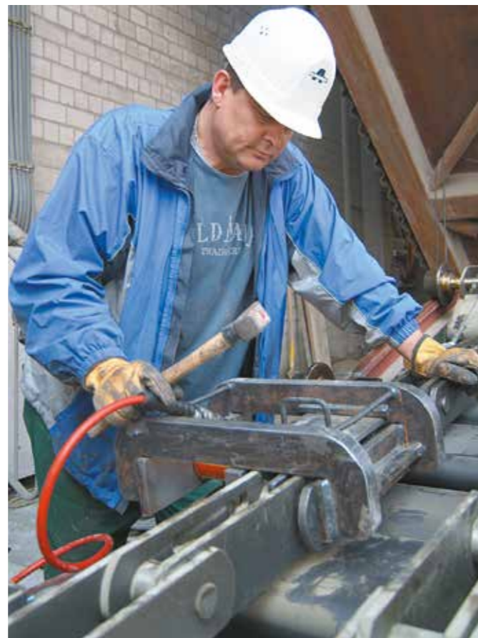
Pre-assembly of chain strands
