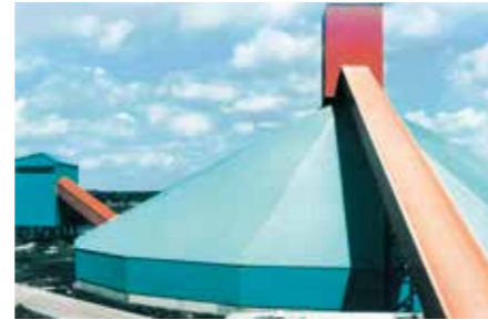
Covered stockpile with MOLEX®
