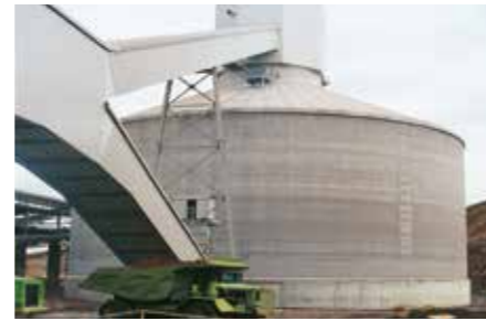
Circular storage hall with internal silo and earth cone
