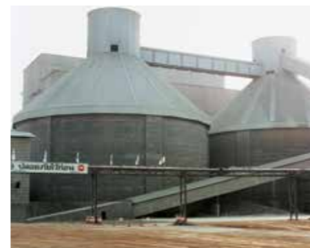
Circular storage hall 2 x 75,000 t
