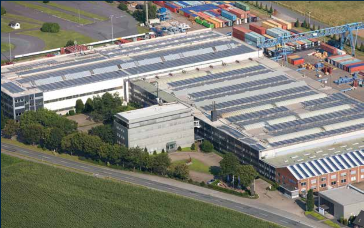
AUMUND headquarters in Rheinberg, Germany
