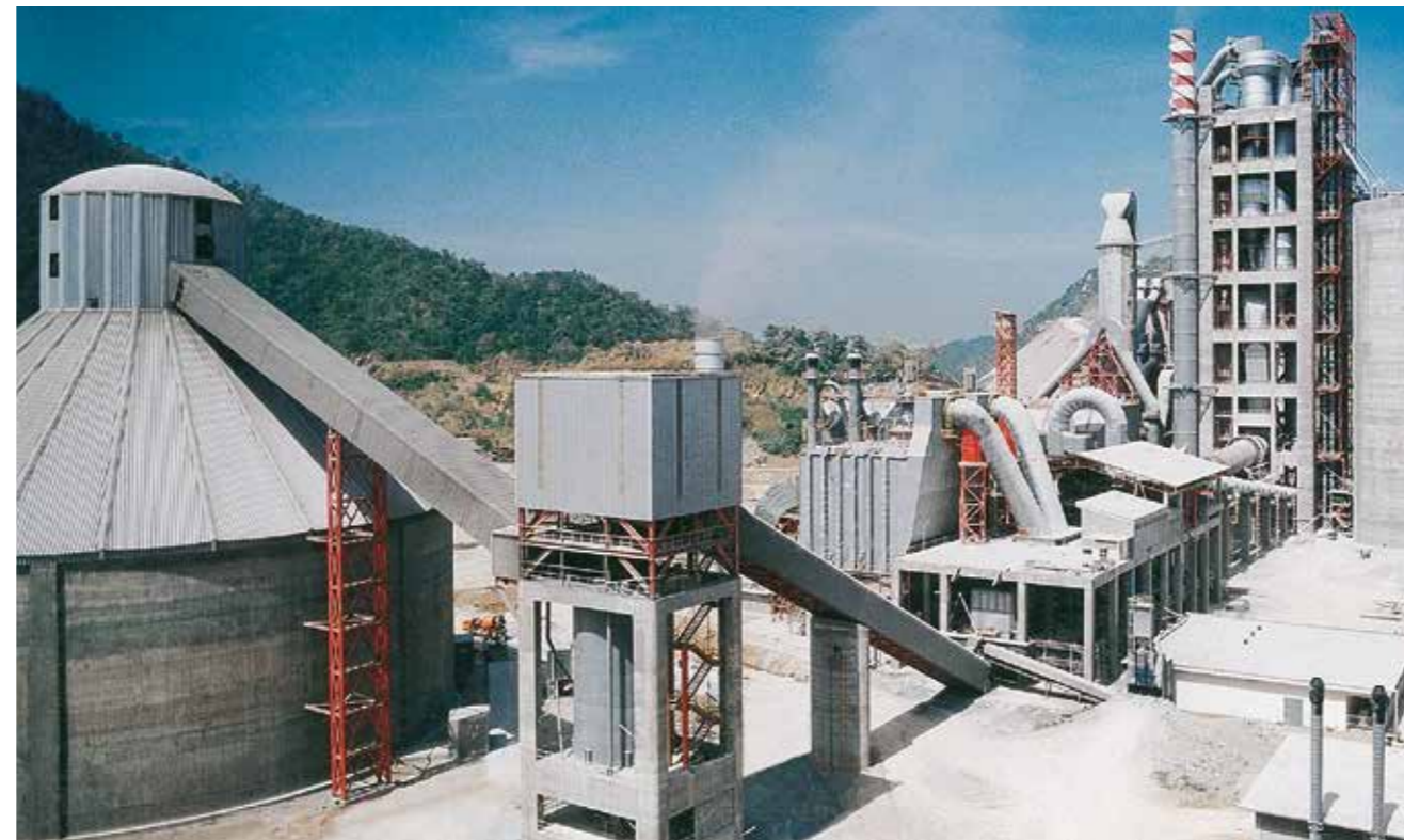
Circular storage hall 150,000 t
