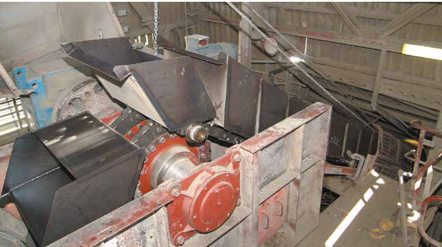
Installation of new bucket strand
