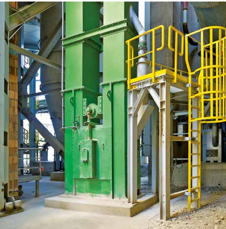
Elevator boot with parallel tensioning device
