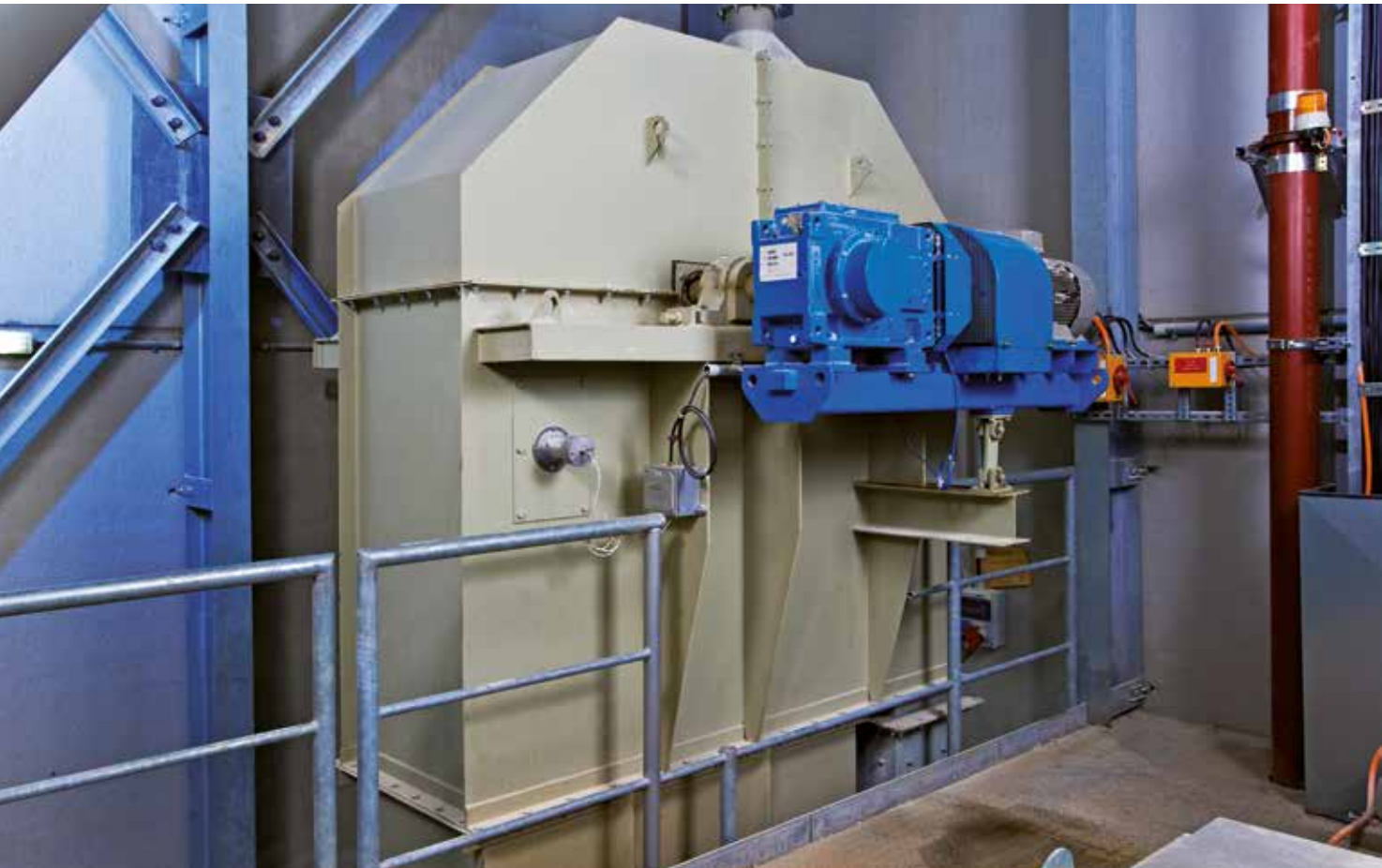
Bucket elevator head with single drive
