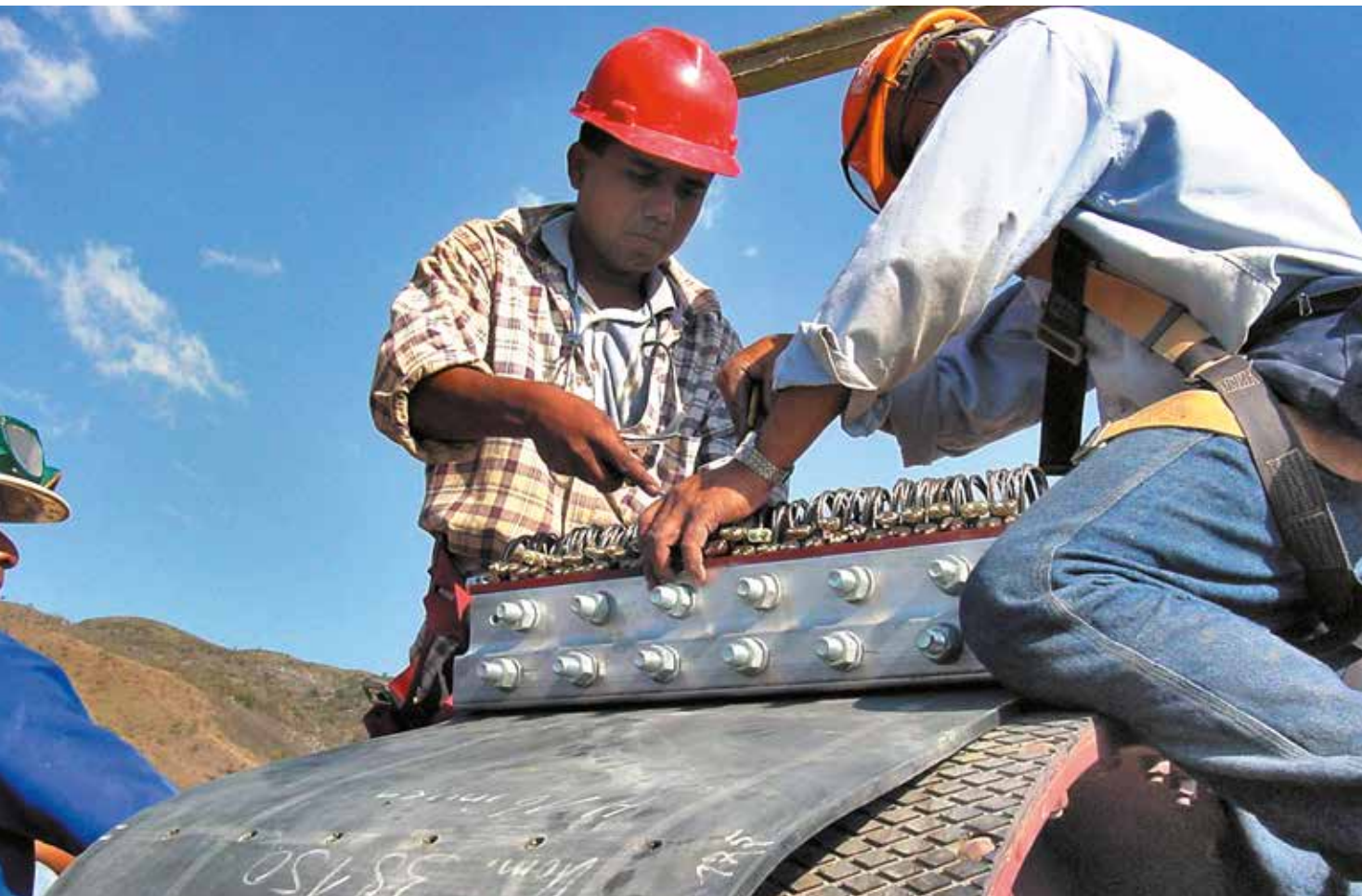
Splicing of steel-reinforced belt
