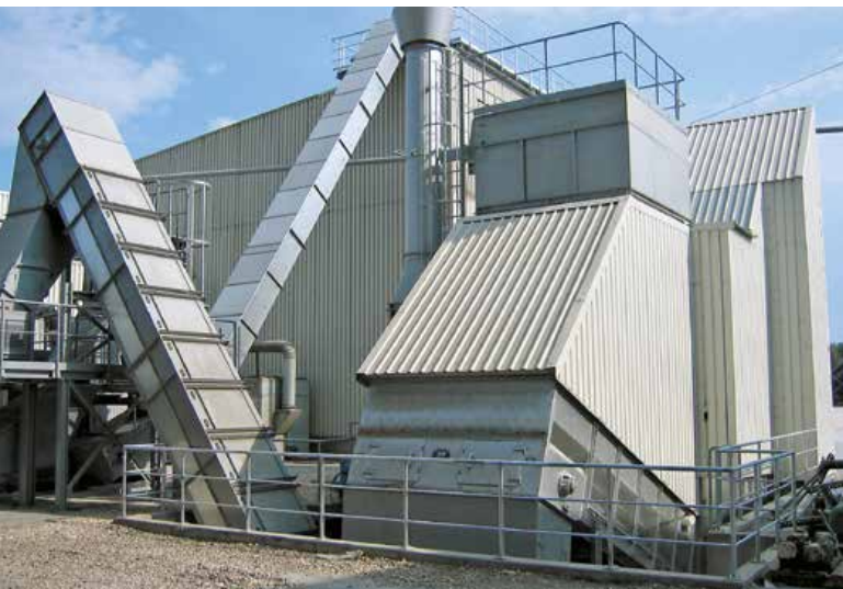
ProFuel intake facility with Drag Chain Conveyor type TKF onward transport
