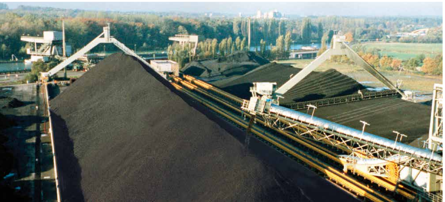
Portal Scraper Reclaimers with Stacker
