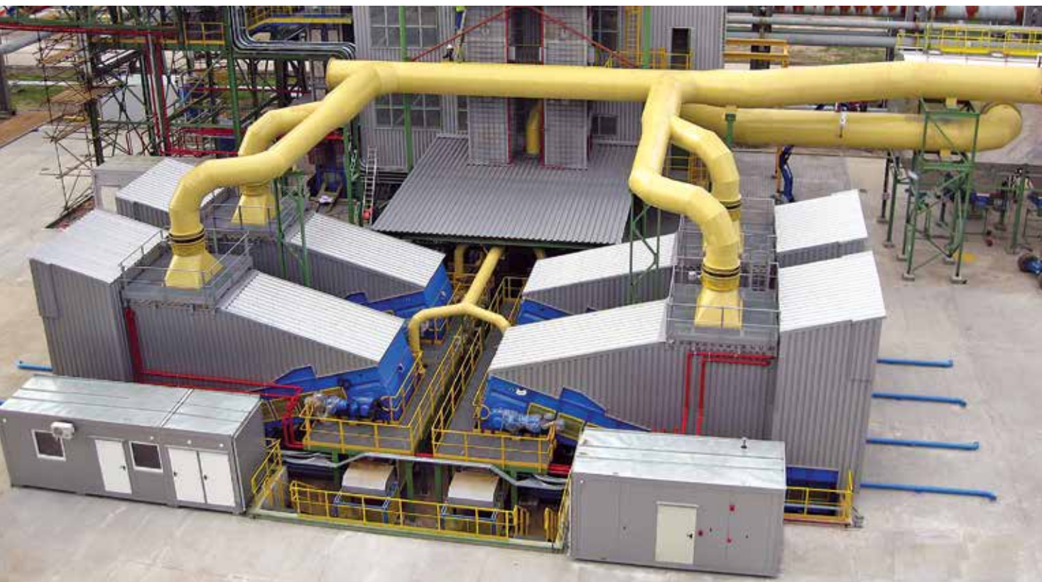
Four Samson® Material Feeders provide an alternative fuel intake facility to a major Power Plant
