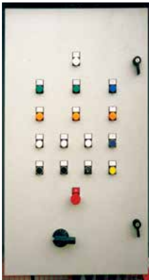
Local cabinet with motor control gear
