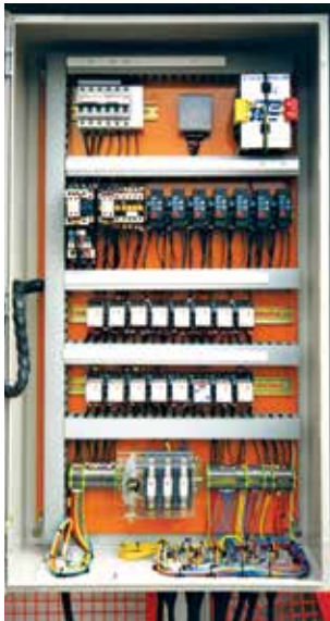
Local cabinet with motor control gear
