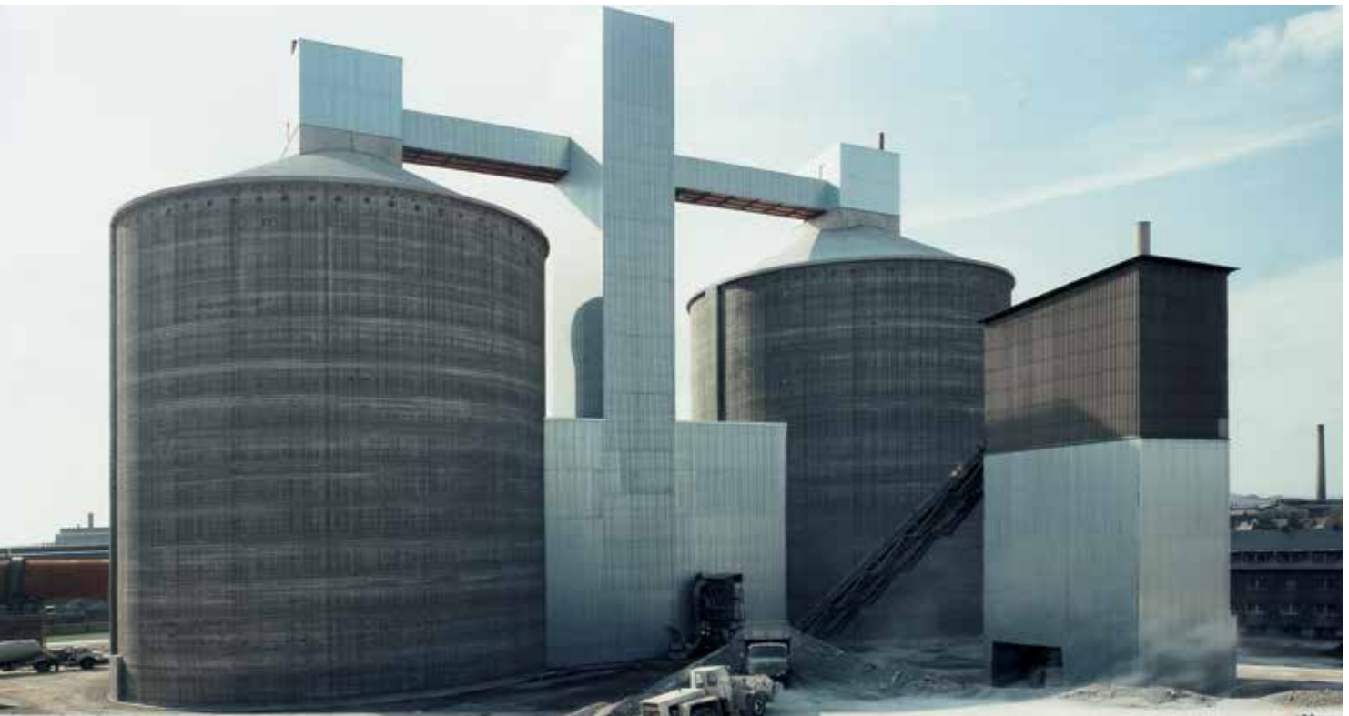
Clinker Silos 2 x 60,000 t (example)
