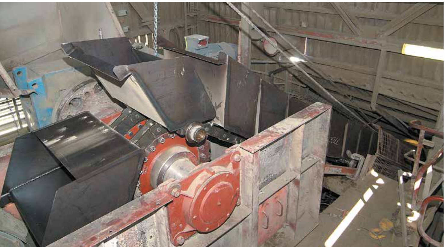
Installation of new bucket strand (example)
