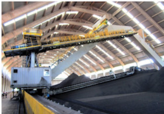
This SCHADE semi-portal reclaimer at Camp Blanco in Ecuador is typical of those installed in China (photo SCHADE)
