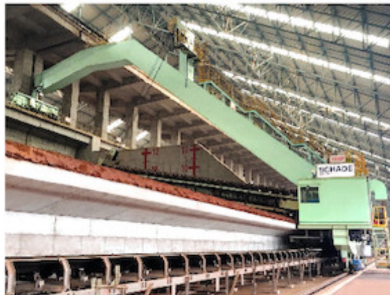
SCHADE Semi-Portal Reclaimer in operation at Baosteel (photo SCHADE)
