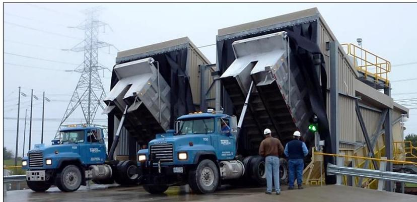
Fig.1. Example for two truck Reception Samson® Material Feeder from AUMUND (showing a similar situation as National Gypsum Shippingport, photo AUMUND)
